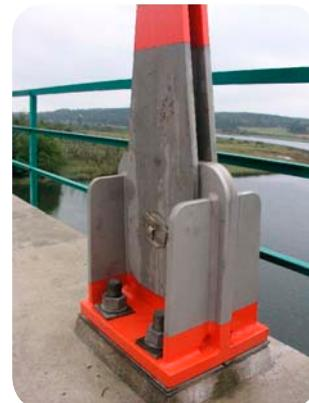
support, which requires very good energy absorbing capability. In a Swedish project one has succeeded in creating a stainless steel bumper support construction that is 26% lighter than the existing structure keeping the costs the same and having the same energy absorbing capacity. The material is HyTens from Outokumpu.
