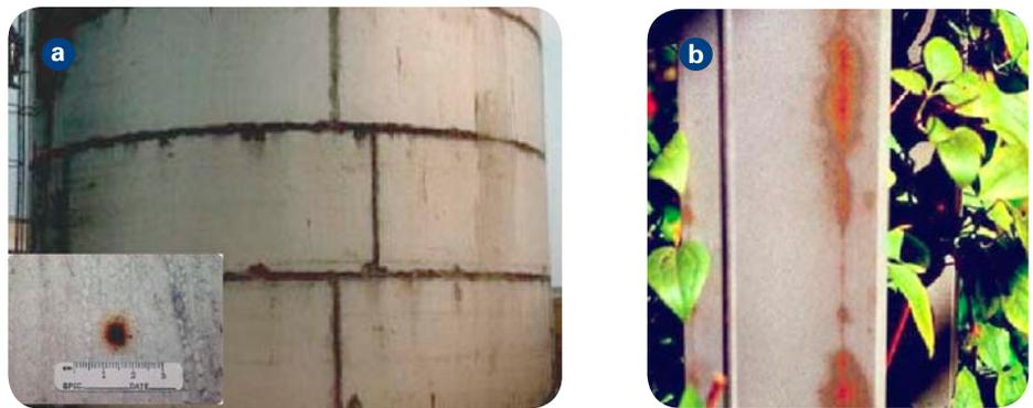
Stress corrosion cracking (SCC) is normally not a problem within the building and construction industry, but one such problem should still be emphasised, SCC in load bearing structures in swimming pool buildings. Volatile compounds, mainly chloramines, can precipitate on cold metal surfaces and cause a special type of SCC, occurring at ambient temperatures.
